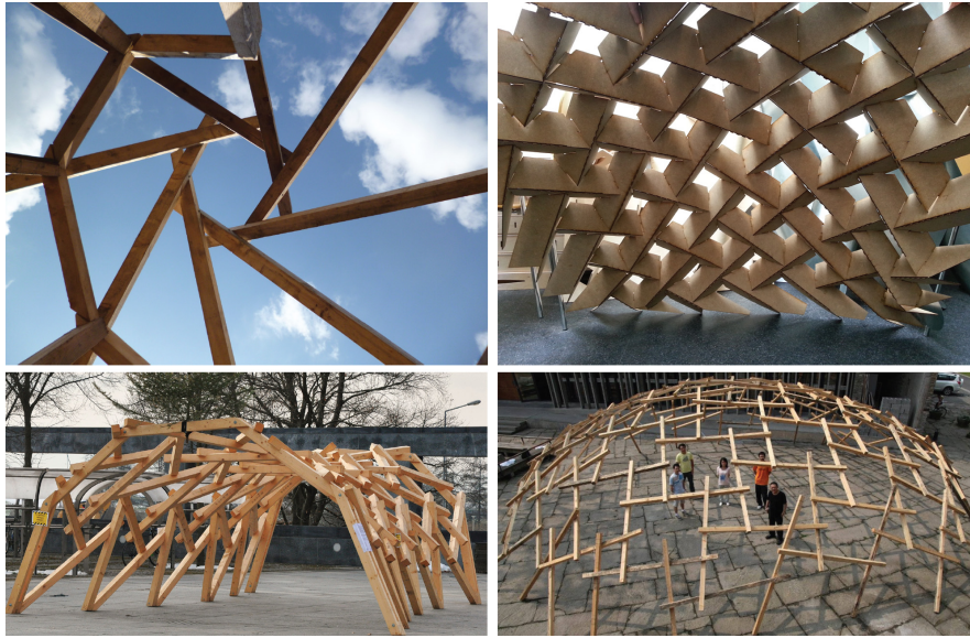
Figure 1: Physical RF-structures designed and fabricated by architects: a simple roof structure (top-left), a design by Michael Clarke (top-right), a design from Spiro-ETH (bottom-left), and a design from Wan Shu and Kengo Kuma (bottom-right).
